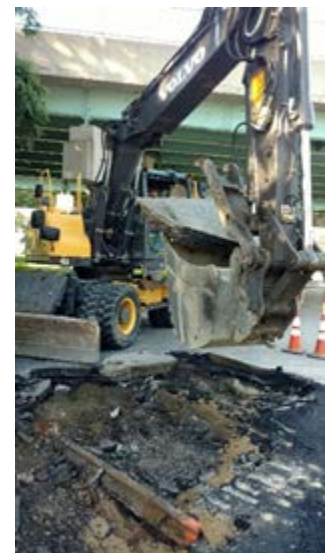
Track Removal Central Avenue at Rutland Street
