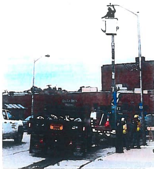
Installation of Affinity LED Lighting in Dover.
