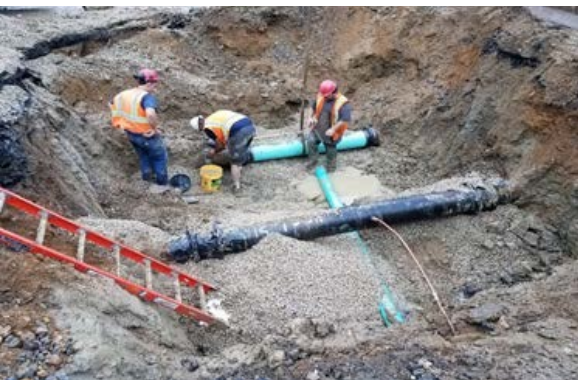
Repairs to Broadway drainline.
