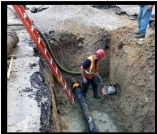
Main Street water main repair.
