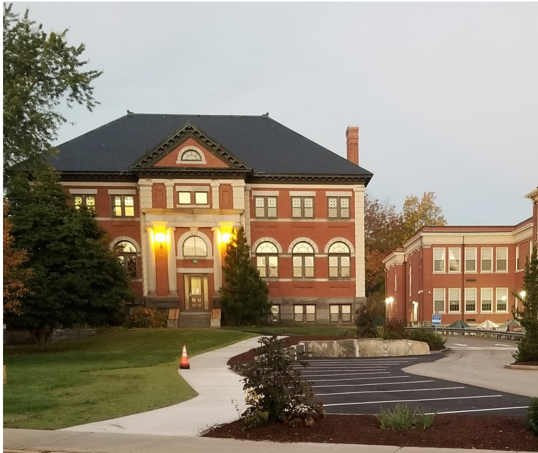
Photo of the new Dover Public Library parking spaces.
