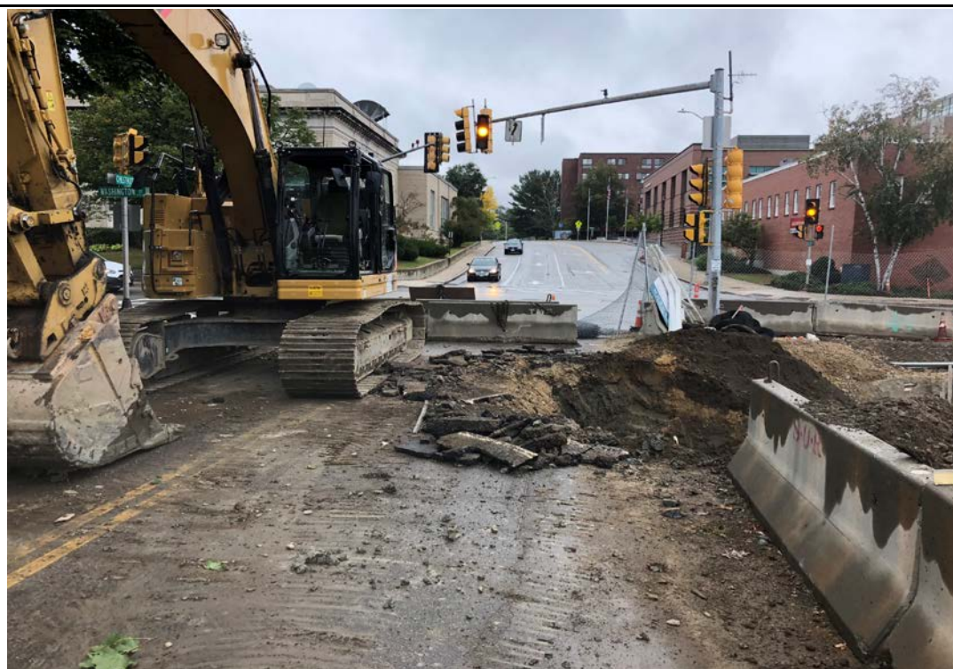
Photograph 6 - View facing north along Chestnut Street showing the extent of impacted soil excavation extending into the Chestnut Street right-of-way. (StoneHill, October 1, 2018)
