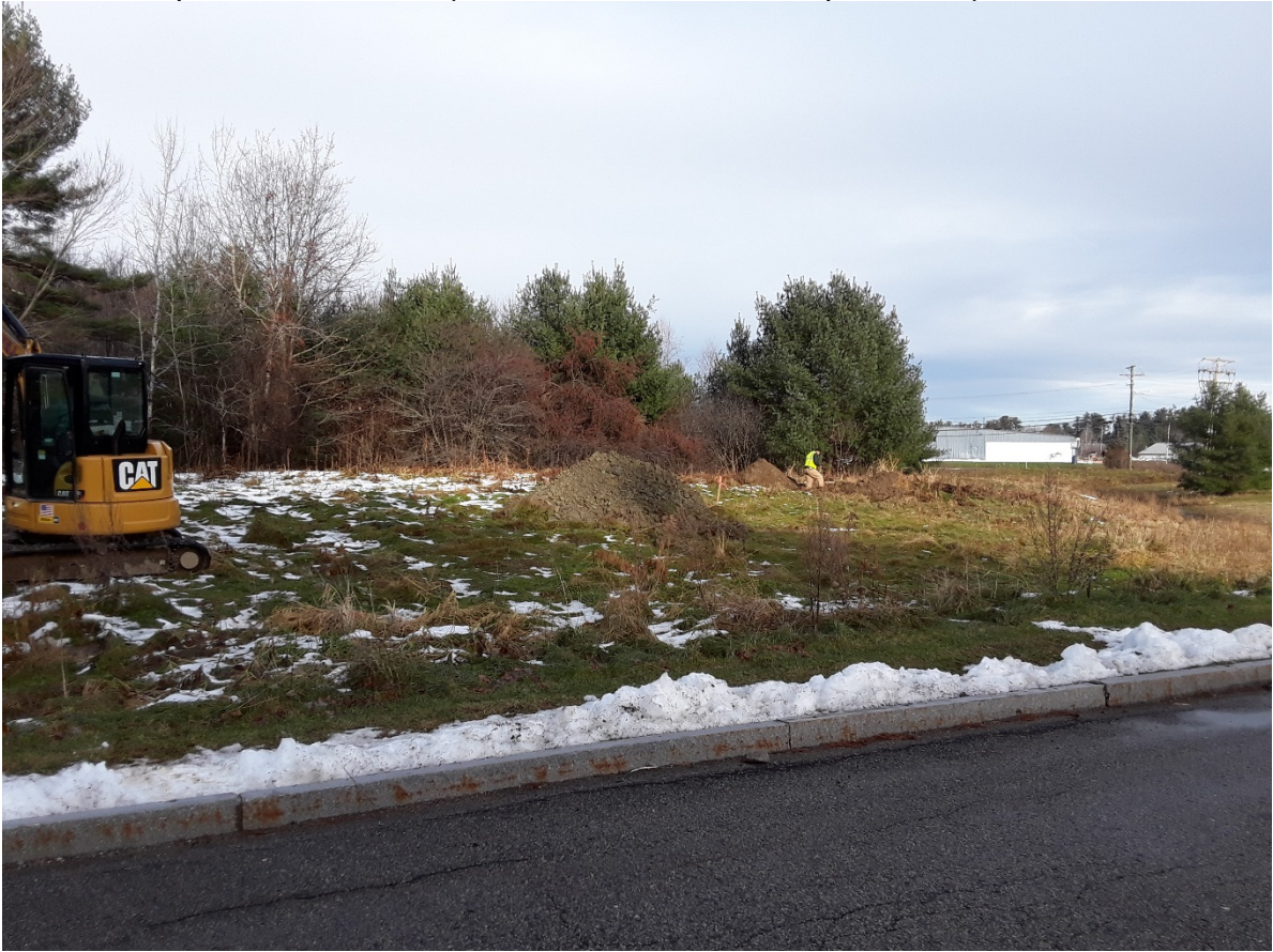
Photo 2: View from Lilac Lane of proposed Lilac Garden residential trash drop-off and compactor site location (see Photo 3 for Trash Compactor Site).
