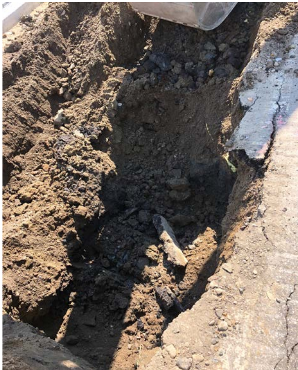
Photograph 4 - View of the extent of UST excavation following tank removal. Two discrete soil samples were collected from the excavation. (StoneHill, September 6, 2018)
