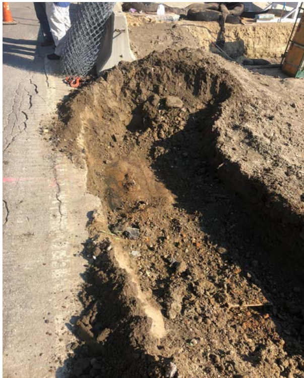
Photograph 2 - View of the top of the tank as it is exposed. No piping was encountered. (StoneHill, September 6, 2018)
