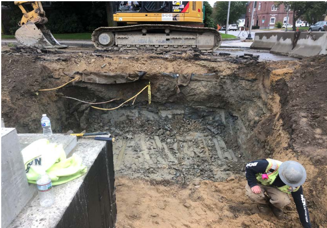
Photograph 5 - View of the extent of impacted soil excavation. (StoneHill, October 1, 2018)
