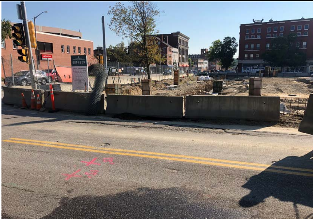
Photograph 1 - View to the east showing Robbins Auto Block construction site east of Chestnut Street. Washington Street is in the background. The UST was located beneath the second from right concrete barrier. (StoneHill, September 6, 2018)
