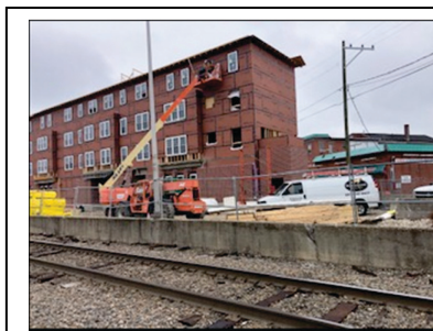
Mixed use building on Third Street.
