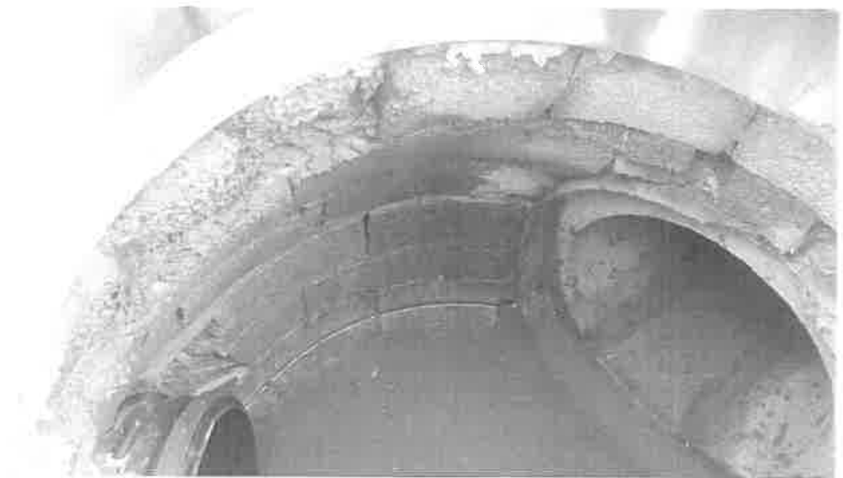
Interior of CB3142
