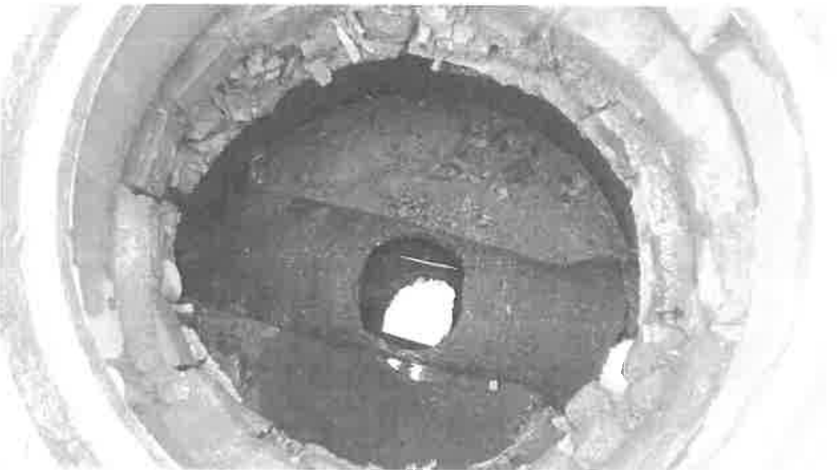
Interior of CB6871
