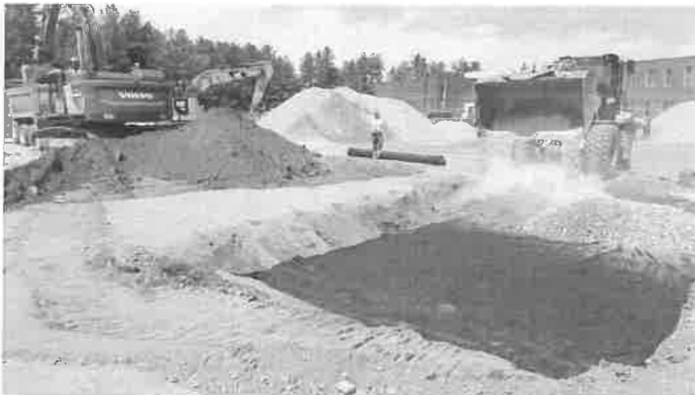
Nonwoven geotextile over clay subgrade, backfill with pavement base course material.
