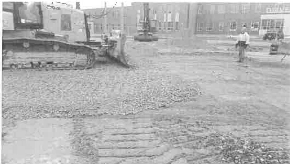
Installation of Base Course on geogrid reinforcement.
