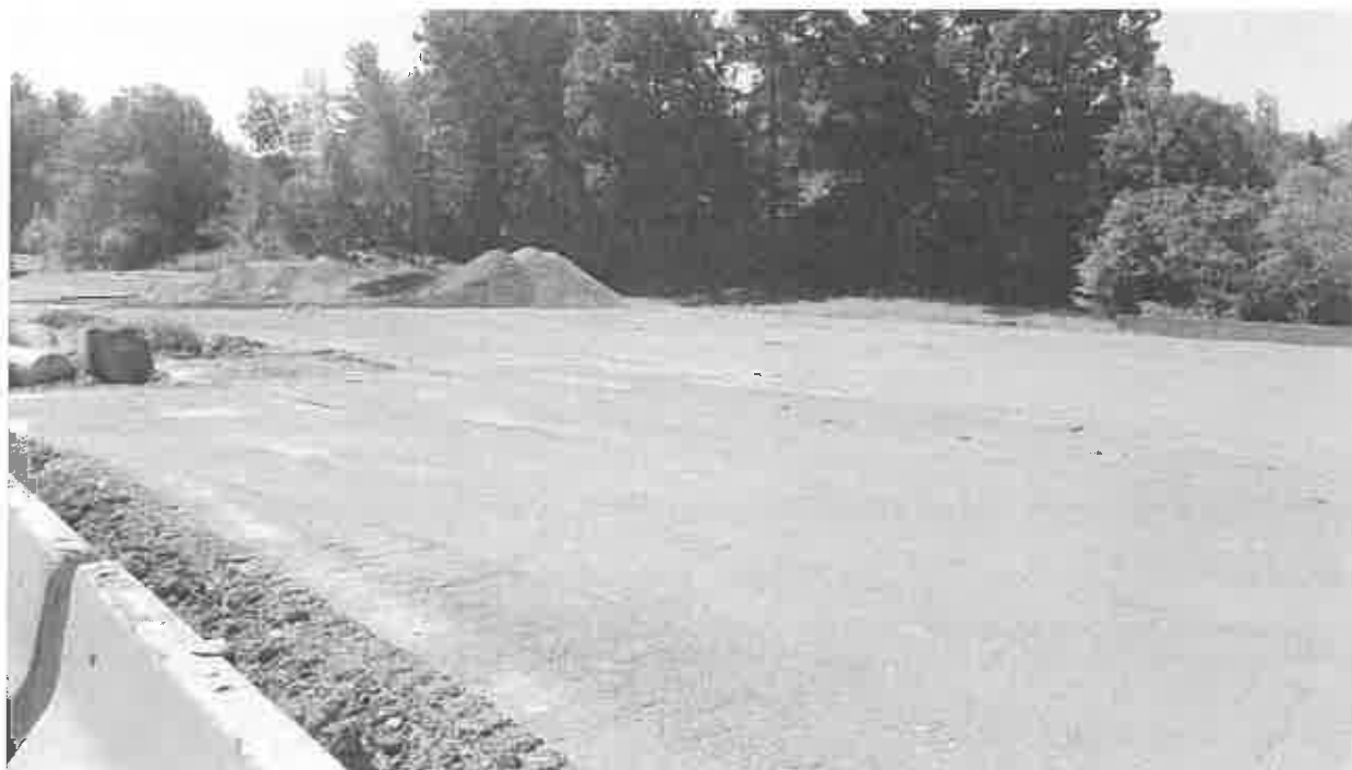
Exposed tennis court subgrade
