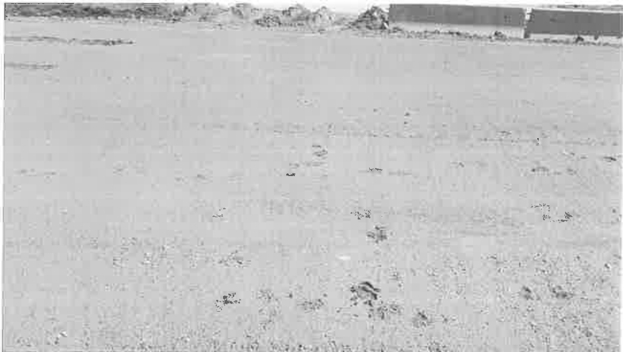
Exposed tennis court subgrade
