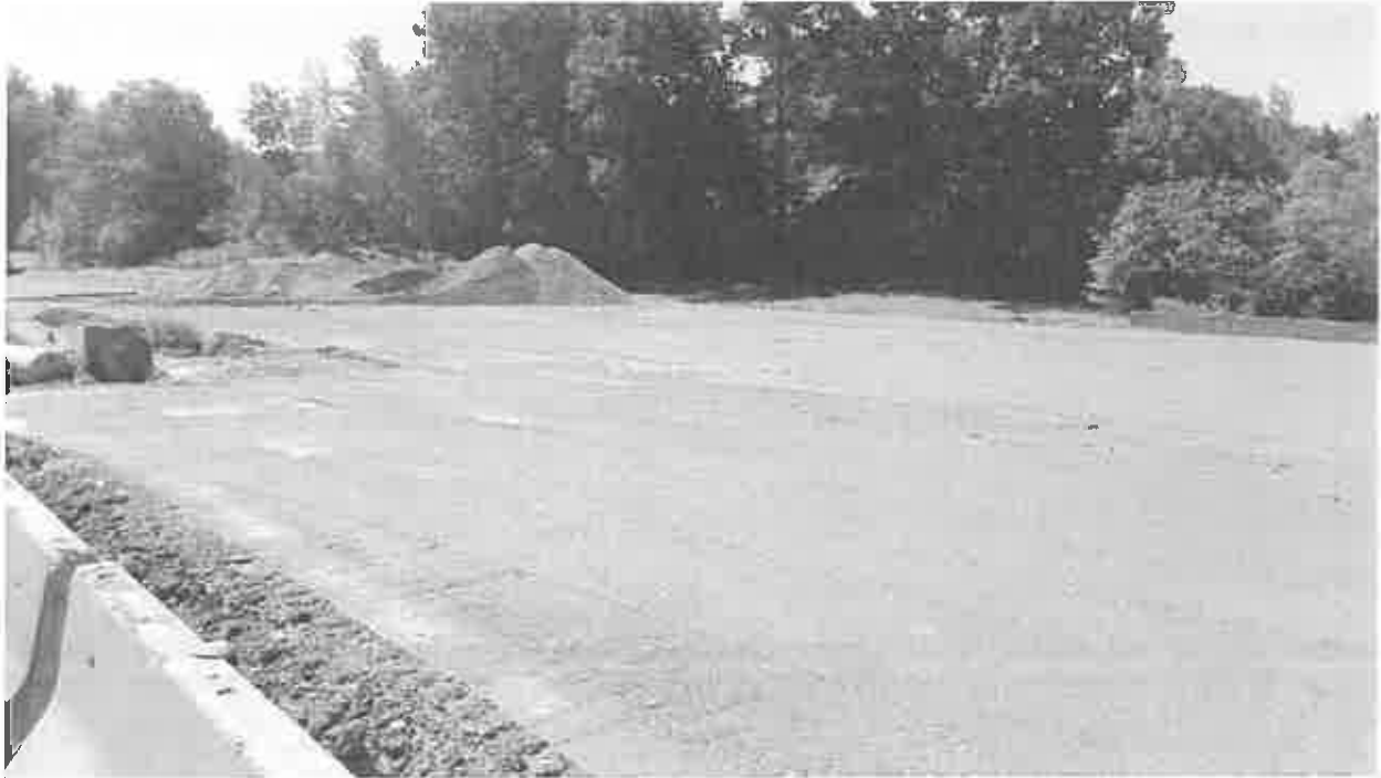
Exposed tennis court subgrade
