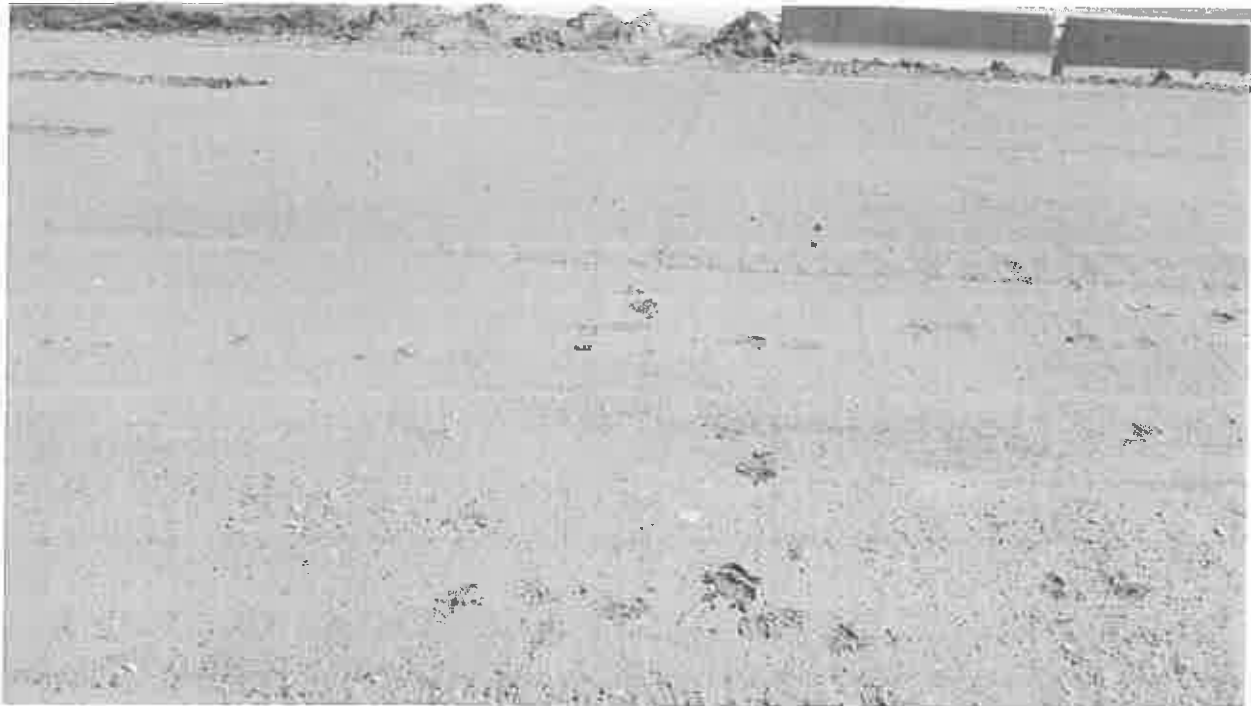
Exposed tennis court subgrade
