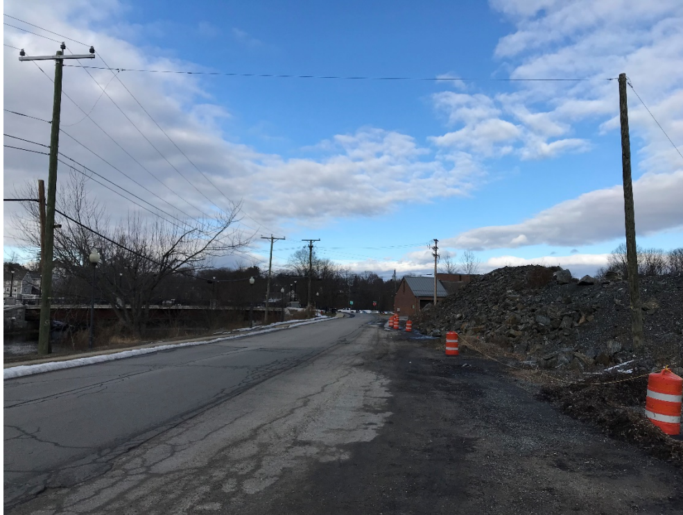
Photo 1: Looking North along River Street
