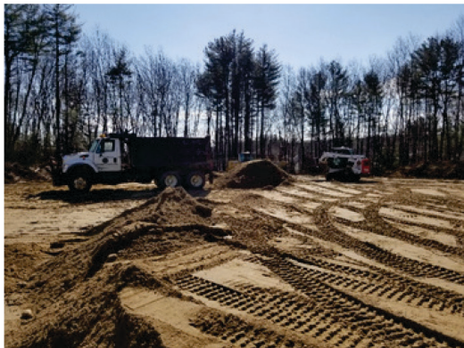
Adding fill to the F&G building site.
