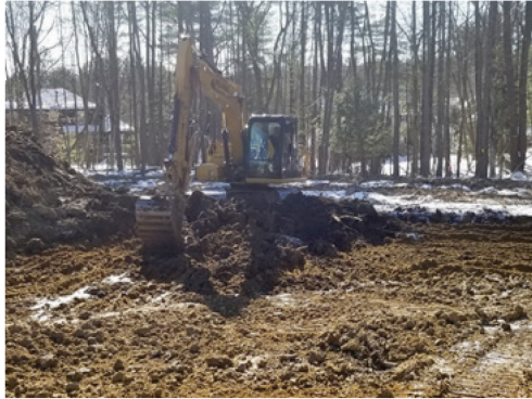
Removing topsoil from the F&G site.
