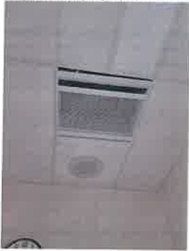
Trainers office, light not secure in ceiling grid. Maybe missing parts
