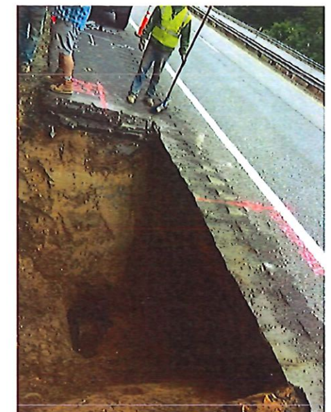
Exposed end of sleeve – Northbound
