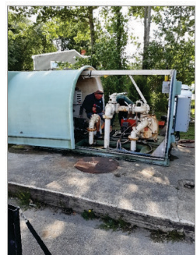
Changeout of pumps at Boston Harbor Pump Station
