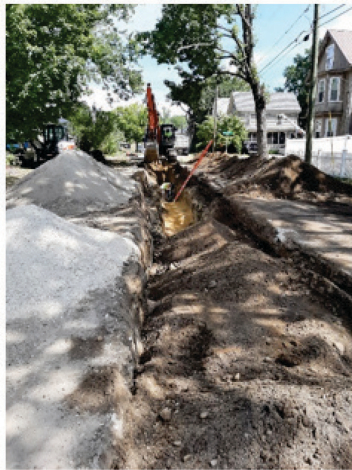
Horne Street pipe installation
